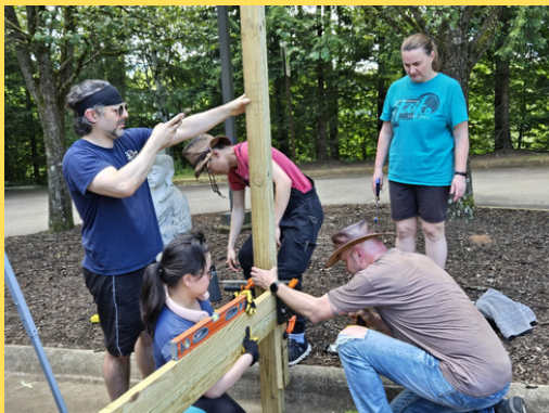
Building a new, bigger, safer Yagura
